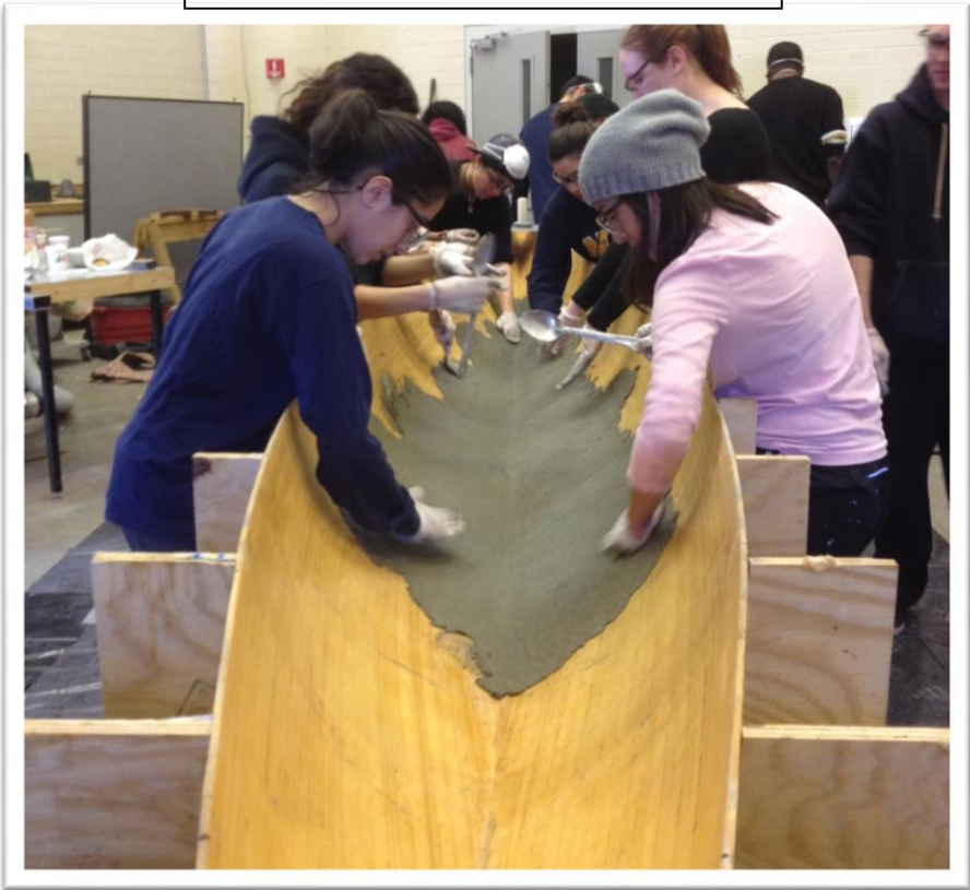
Photo 4: First Layer of Concrete
