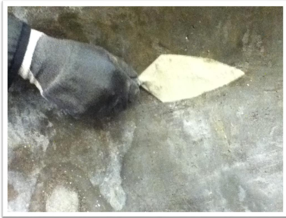
Photo 1: Patching Along Inside of
