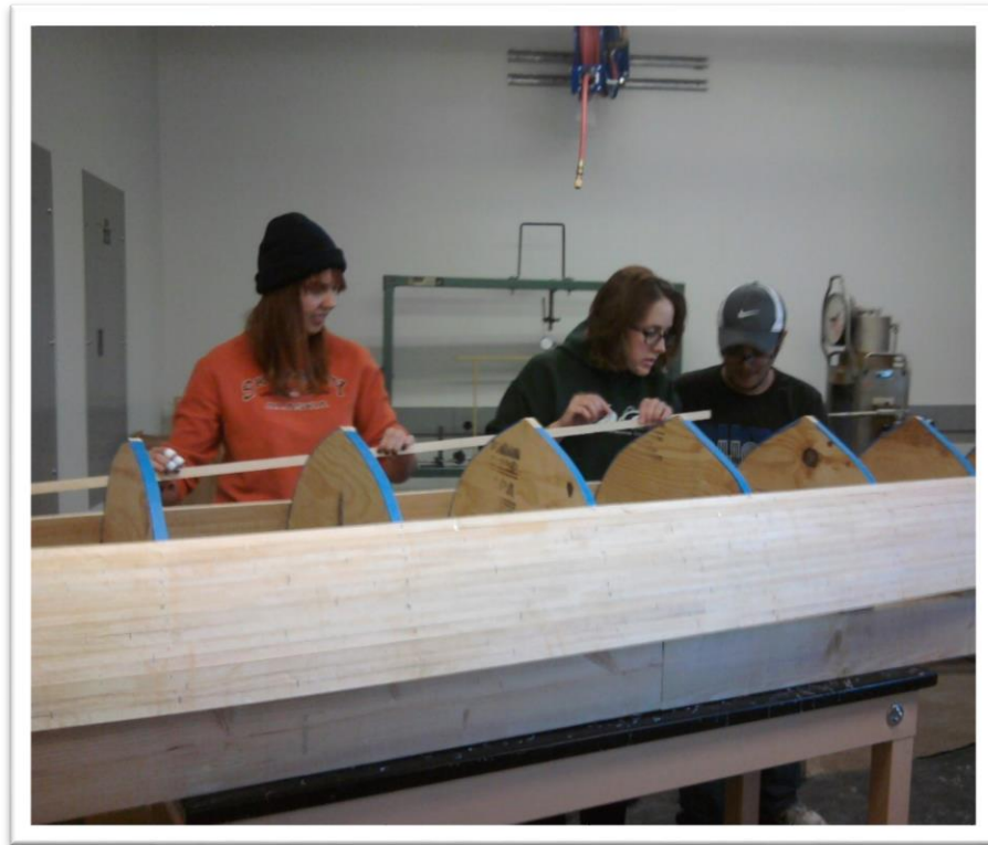
Photo 3: Attaching Wood Strips to Cross-
