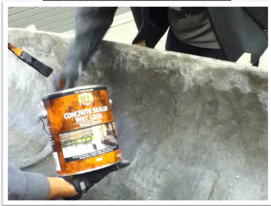
Photo 4: Application of Concrete
