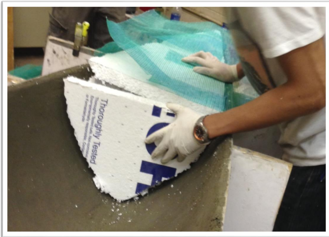
Photo 7: Installation of Foam
