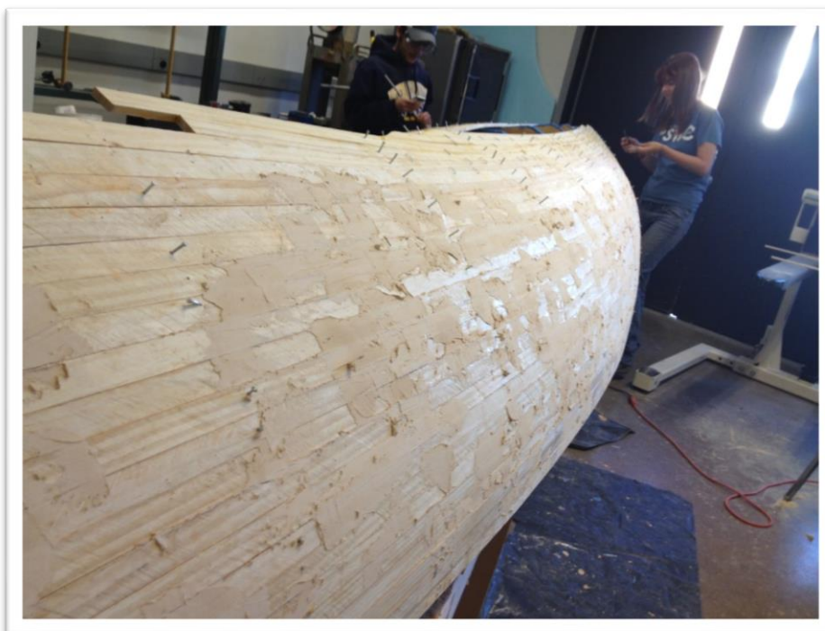
Photo 5: Patching Holes in Wood
