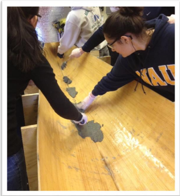
Photo 1: Form Oil and First Layer of Concrete
